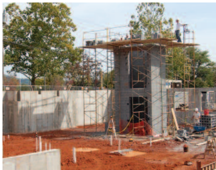
Elevator shaft being built in Apartment-Condo building.
